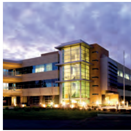
8 Facade and Exterior Lighting
